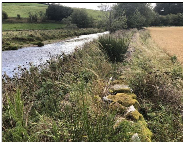
Figure 3.4. Example of the stone wall along the top of the River Don right bank, limiting channel floodplain connectivity.
