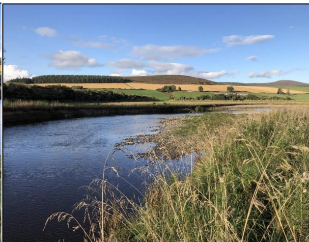
Figure 3.8 Looking across the channel to the embankment breach area on the river left bank.
