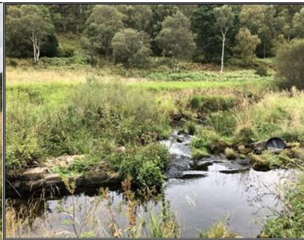
Figure 3.32. Partially intact boulder weir located at OS NGR NJ 48849 18692.
