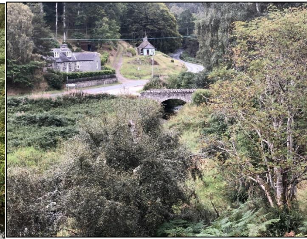
Figure 3.36. Arch bridge providing vehicular access to the Ardhuncart Estate. This bridge is positioned ~80 m upstream from the Mossat-Don confluence OS NGR NJ 49038 18555.
