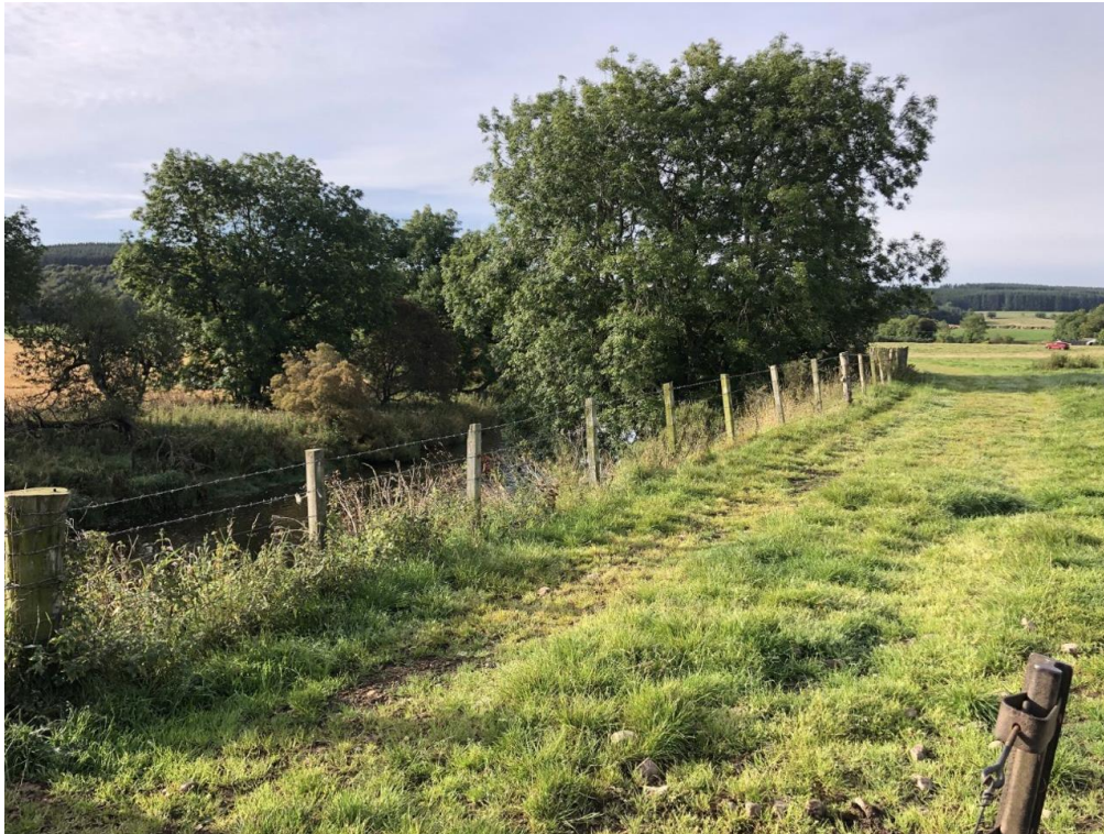
Figure 4.19 Fence line positioned along the top of the River Don right bank, next to Jock Reid pool. This section of bank is just upstream of the bank erosion and embankment breach. Recommend to set-back the fence line and reprofile the bank, to provide long-term bank stability.
