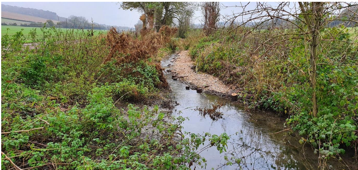
Figure 4.11 Example of an in-channel bench constructed on the right bank of this river. The top of the brushwood with chestnut stakes, forming the outer edge of the bench can just be seen above the water surface.
