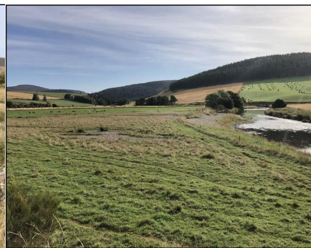
Figure 3.12. Embankment breach area. Continuous tree line on the top left of this photo shows the position of the Auld Water.
