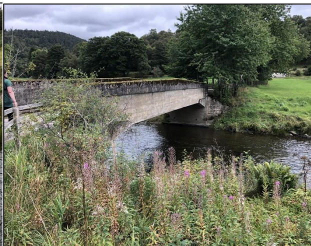
Figure 3.20 Bridge between Delphorrie and Macharshaugh.
