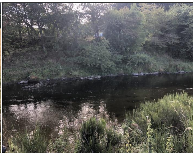
Figure 3.5. Stone toe protection present intermittently throughout. Photo shows a section of river left bank protection downstream of Cleek-Him-In-Pot pool.
