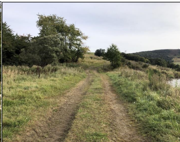
Figure 3.26. Track over the Auld Water, ~10 m upstream from the Don confluence. The channel passes through a culvert at this point.
