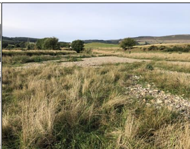
Figure 3.11. Cobble, gravel and fine sediment deposited on the floodplain within the embankment breach area.
