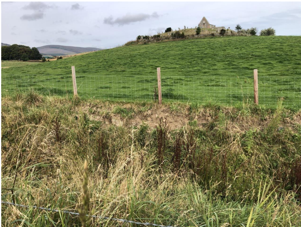
Figure 4.21 Bank erosion observed on the river left bank within the same field as St. Brides Chapel. The fence line along the top of bank here is likely to be undermined in future flood events when this bank is subject to further erosion.
