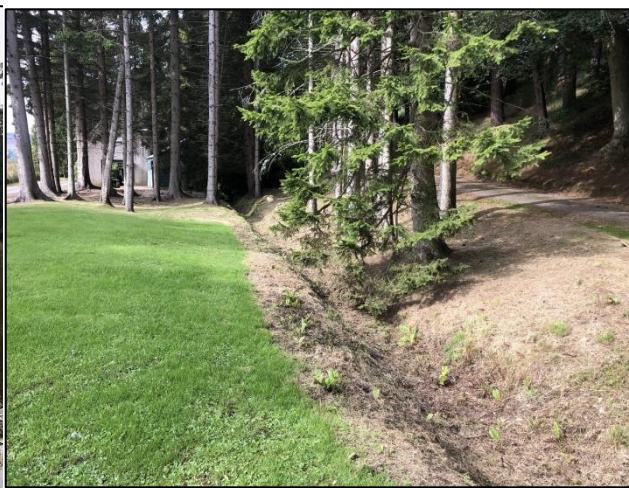
Figure 3.17. Drainage ditch between the road to Ardhuncart Lodge and the Gardener's Cottage garage.
